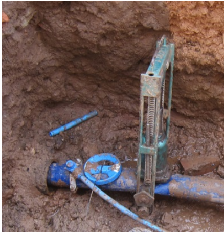
The left image shows a tagged ferrule & squeeze-off point, whilst the right image shows a tagged split on a customer pipe - a potential point for future background leakage due to the excessive use of push-fit joints
